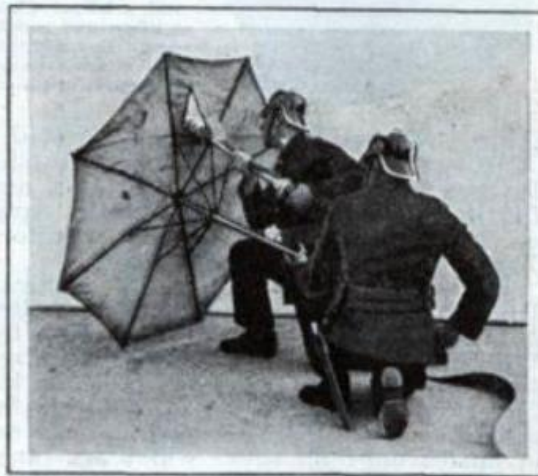
This large type of asbestos umbrella permits several hose nozzles to be thrust through it, protecting firemen from heat.
