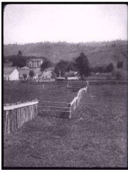
This picture, taken near Bolinas in Marin County by G.K. Gilbert, shows a fence that was offset about 8.5 feet along the trace of the fault (from Steinbrugge Collection of the UC Berkeley Earthquake Engineering Research Center)
