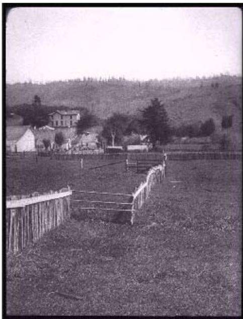
This picture, taken near Bolinas in Marin County by G.K. Gilbert, shows a fence that was offset about 8.5 feet along the trace of the fault (from Steinbrugge Collection of the UC Berkeley Earthquake Engineering Research Center)
